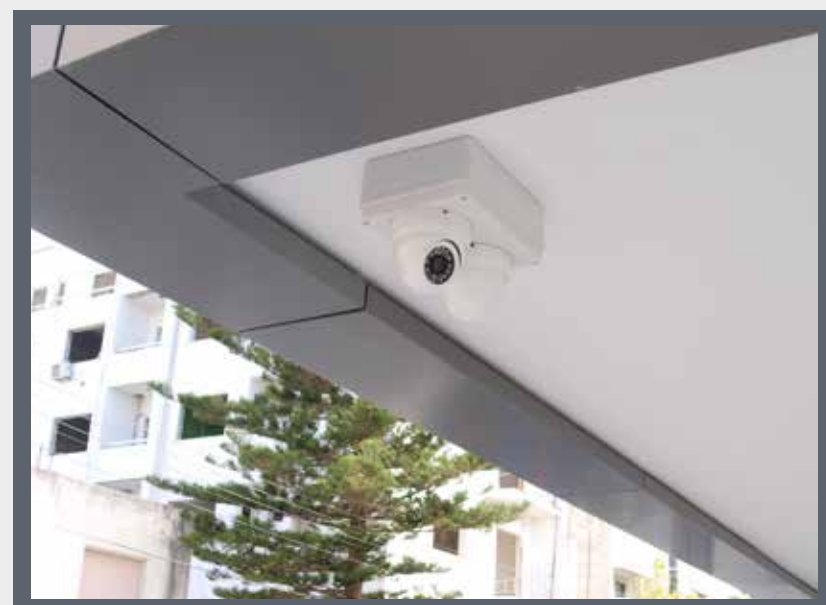
CCTV FOR ALL COMMON AREAS
